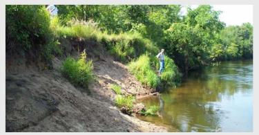
Root wads were used to stabilize two sites on the Rum River in Anoka, Minnesota, where severe bank erosion threatened to destroy adjacent trails. Approximately six root wads were placed at each site under difficult, high-water conditions. The banks were then graded, topsoil was added, and native vegetation was planted. Despite the difficult placement, the root wads have protected the lower bank, allowing the vegetation to become well established.
