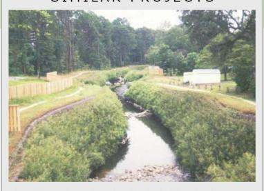
The Mill Creek Restoration Project utilized soil bioengineering design to stabilize 175 linear feet of severely eroding streambanks within the Caldwell Recreation Park in southeastern Ohio. The work included two 25-foot vegetated reinforced soil slope (VRSS) sections, two 50-foot fill bank sections protected with woven coir and direct woody plantings, and a 12.5-foot tie-in on the upstream and downstream end of streambank work area.
