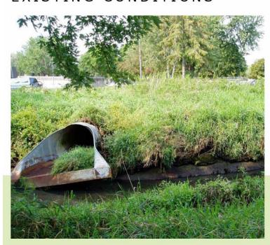
Erosion is frequently observed at culvert outlets for a variety of reasons, including insufficient erosion protection at the culvert outlet, streambank erosion, and channel downcutting, which leaves the culvert perched above the channel. Filter fabric is often used at culvert outlets to separate riprap protection from underlying soils, however the fabric provides a slippery surface for the riprap, which commonly slides into the channel.
