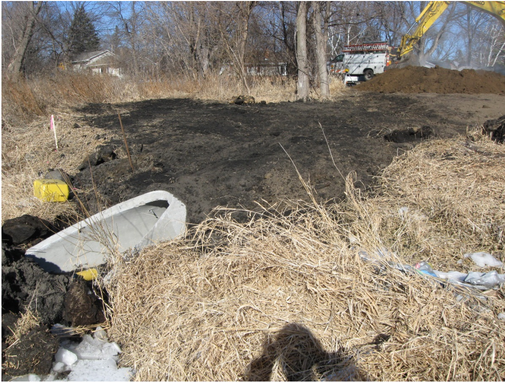
Installation of outlet pipe to Bassett Creek
