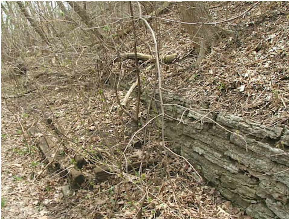
Photo 8: Bassett Creek Park Retaining Walls (detail).
