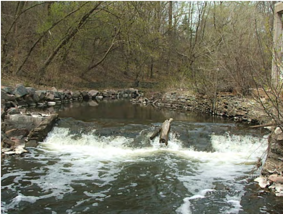
Photo 4: Dam - Note Rip Rap (left) and Stone Walls (right).
