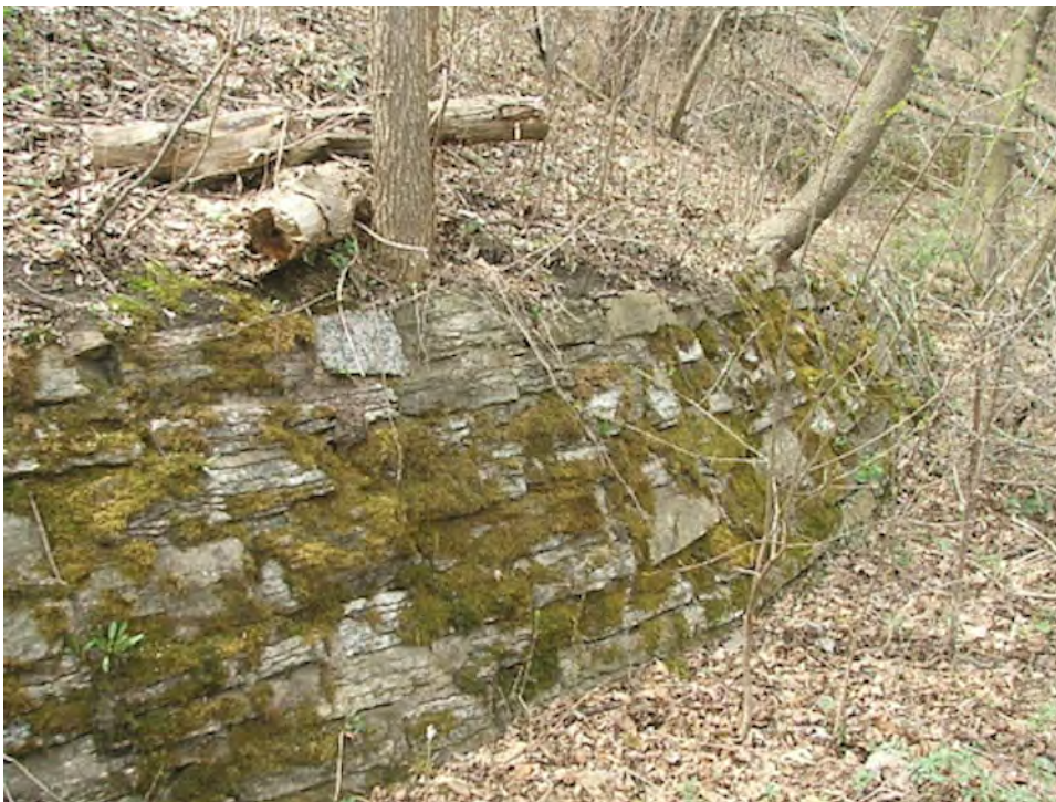
Photo 12: Bassett Creek Park Retaining Wall (detail).
