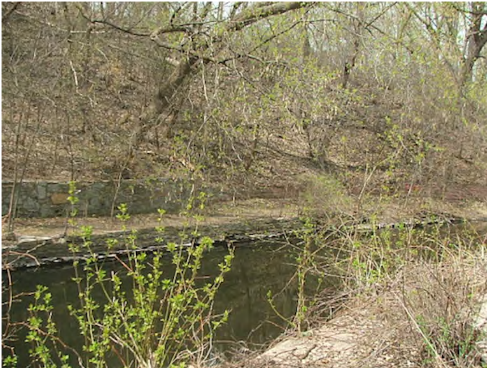
Photo 4: Bassett Creek Park Stone and Brick Retaining Walls.
