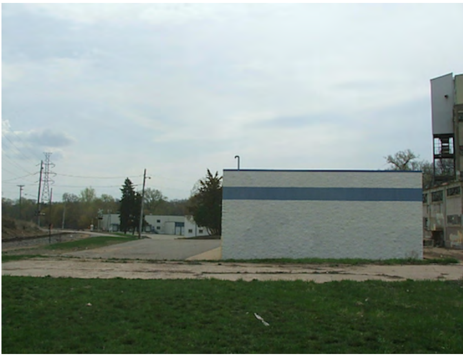
Photo 1: Glenwood-Inglewood Water Company.
