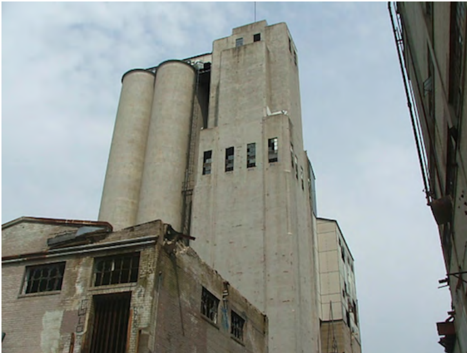
Photo 6: Fruen Mill Grain Silos and Elevator.
