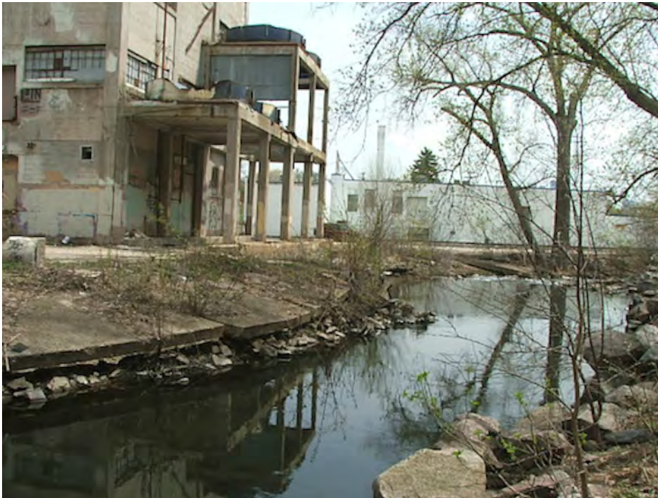
Photo 12: Downstream toward dam, Fruen Mill (right), and Glenwood-Inglewood Water Company (background).
