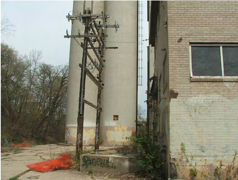
Photo 11: Fruen Mill Power Poles and Silos.
