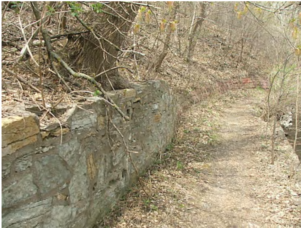
Photo 2: Bassett Creek Park Retaining Walls.
