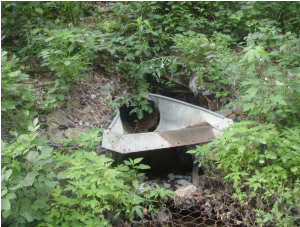
Photo 14. Site 9. Erosion around flared end section.
