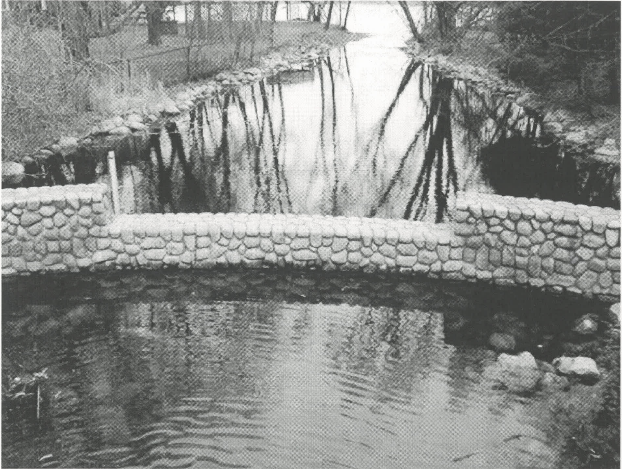
Photo 2: Channel approach fills to dam one day after ice out. Notice how area below the dam is also filled with water. No water appeared on either side of dam as late as March 17, 2012. Photo taken March 19, 2012.
