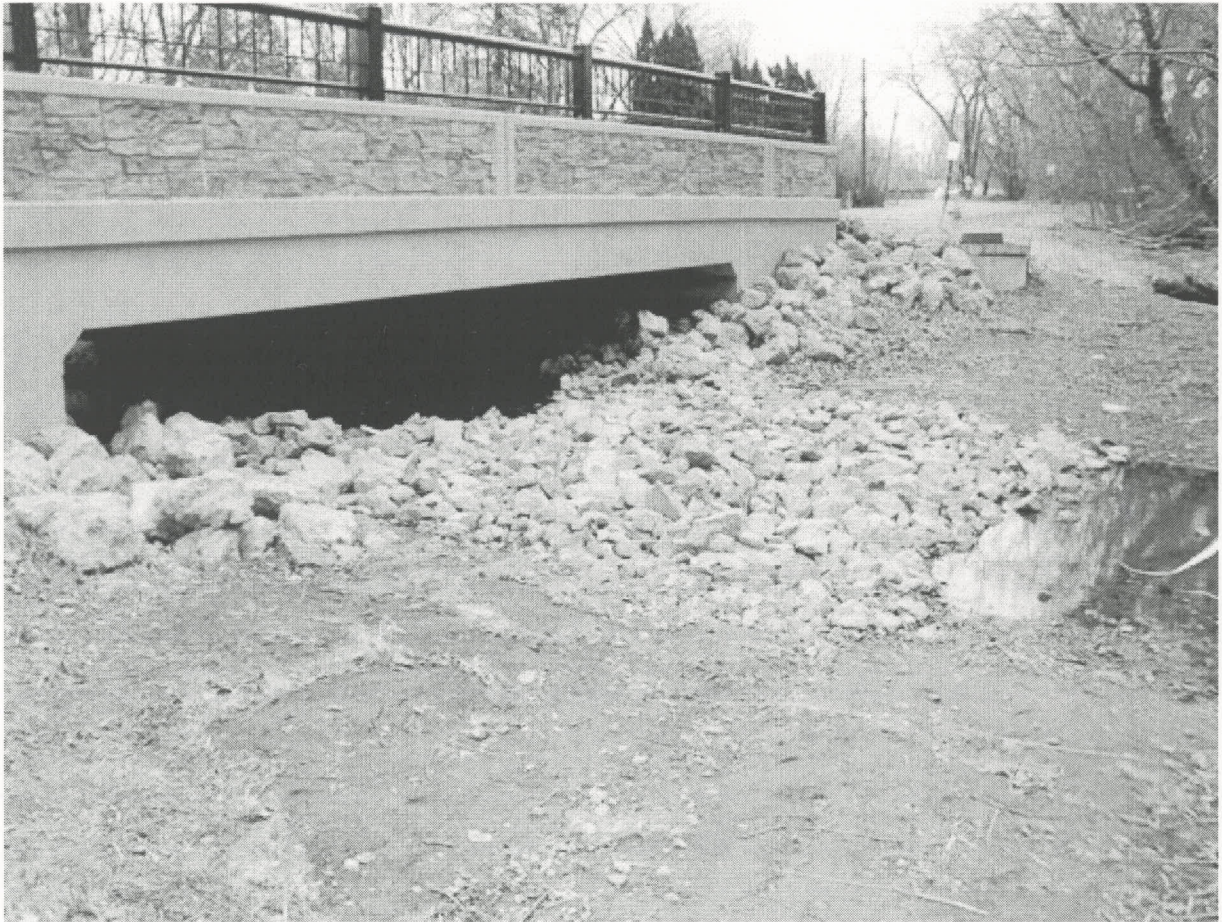
Photo 5: South side of bridge showing creek bed with new granite riprap placed over sanitary sewer line. Notice the amount of constriction in opening under the bridge. Photo taken March 19, 2012.
