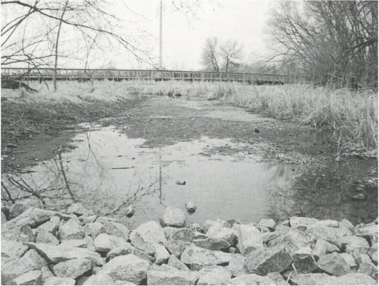
Photo 7: View looking south down creek from atop newly placed granite riprap. Notice some water is leaking through riprap obstruction and is flowing into creek. Photo taken March 19, 2012.
