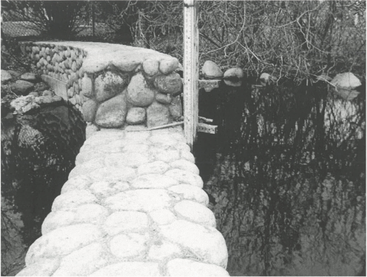
Photo 3: View of weir and lake level measuring gage. Notice that lake water level is about two to three inches short of cresting over the weir. Photo taken March 19, 2012.
