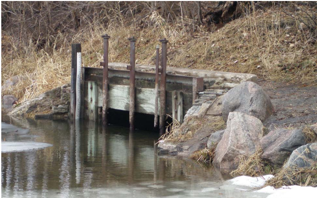
Figure 2. Existing Wirth Lake Outlet Structure.
