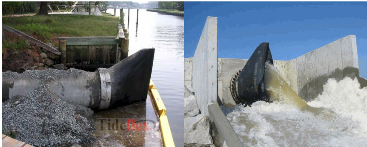
Figure 4. Photos of the Rubber Check Valve.
