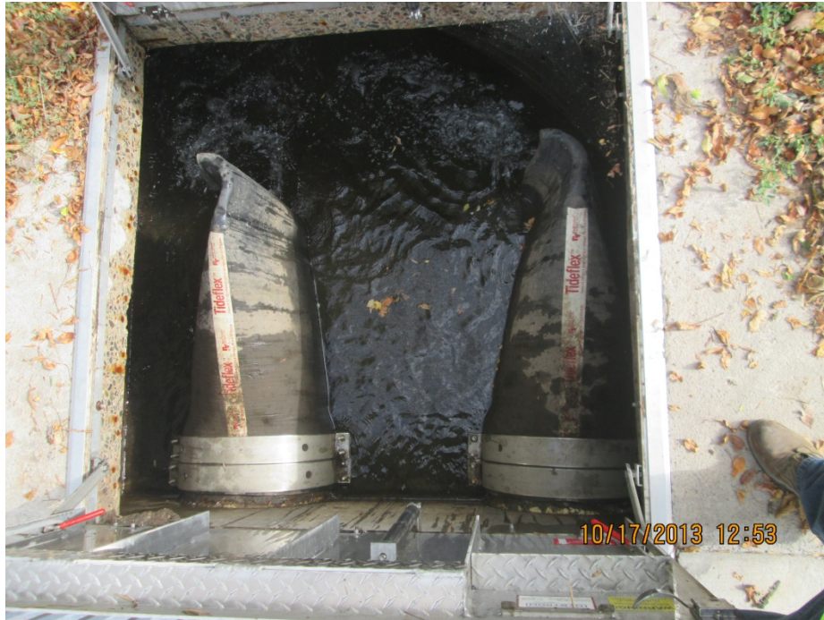
Rubber check valves installed inside new outlet structure, October 2013
