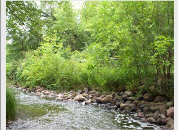
Stone toe protection has been used extensively in Nine Mile Creek's Lower Valley, in conjunction with deflector dikes, grade control measures and stabilization of large bank failures. Following the 1987 "super storm," the proposed design allowed the stream to continue its course while taking measures to protect areas where water flow was eroding valley walls. The resulting measures have stabilized the stream channel and valley walls while blending seamlessly with the natural environment.
