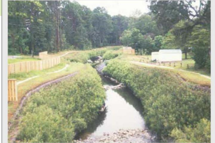
The Mill Creek Restoration Project utilized soil bioengineering design to stabilize 175 linear feet of severely eroding streambanks within the Caldwell Recreation Park in southeastern Ohio. The work included two 25-foot vegetated reinforced soil slope (VRSS) sections, two 50-foot fill bank sections protected with woven coir and direct woody plantings, and a 12.5-foot tie-in on the upstream and downstream end of streambank work area.
