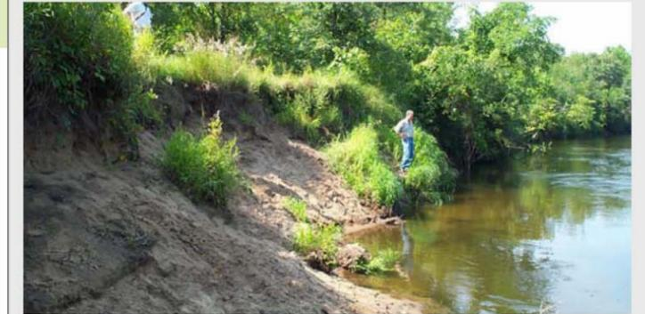
Root wads were used to stabilize two sites on the Rum River in Anoka, Minnesota, where severe bank erosion threatened to destroy adjacent trails. Approximately six root wads were placed at each site under difficult, high-water conditions. The banks were then graded, topsoil was added, and native vegetation was planted. Despite the difficult placement, the root wads have protected the lower bank, allowing the vegetation to become well established.
