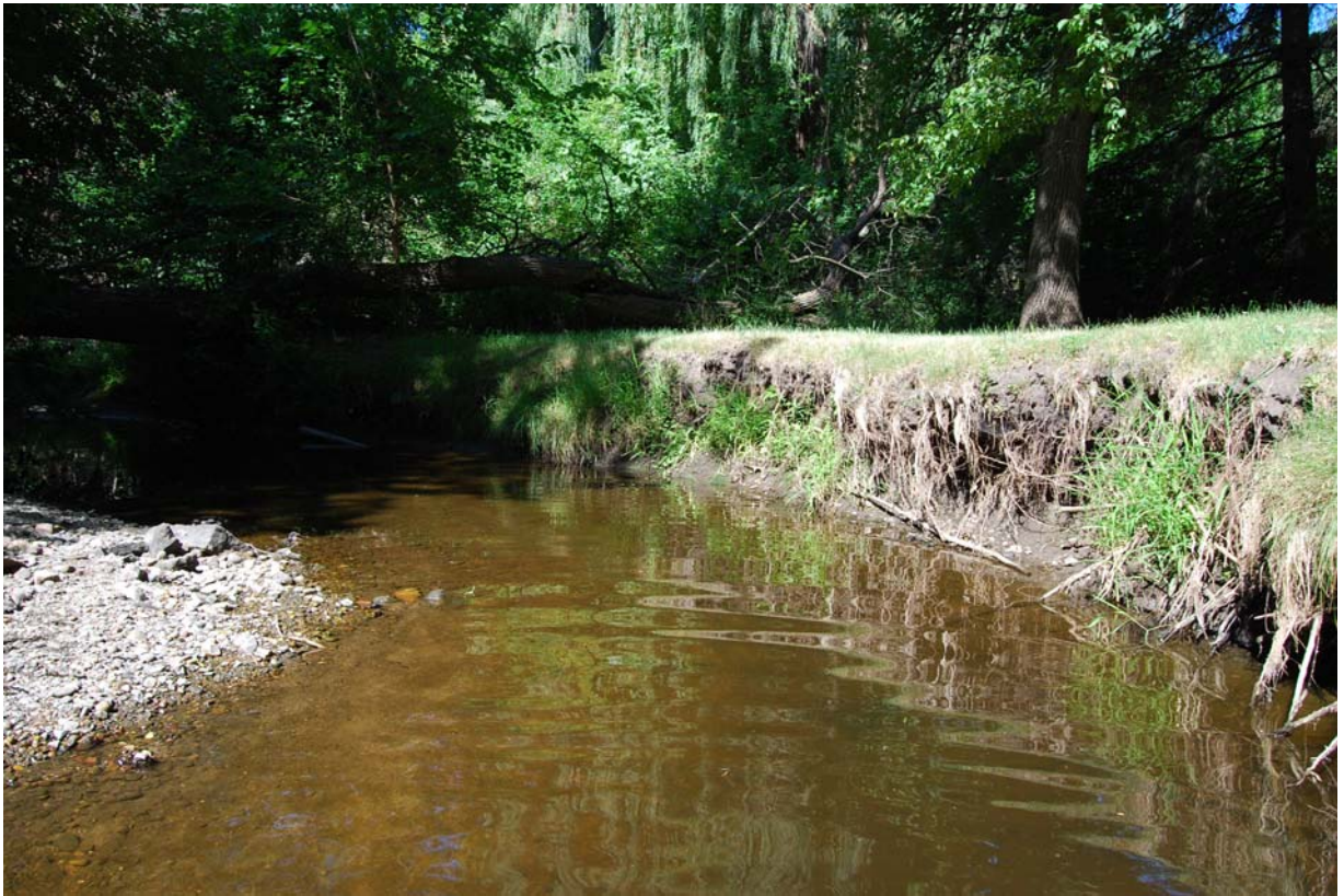
Stream bank erosion and existing vegetation at Site 5.
