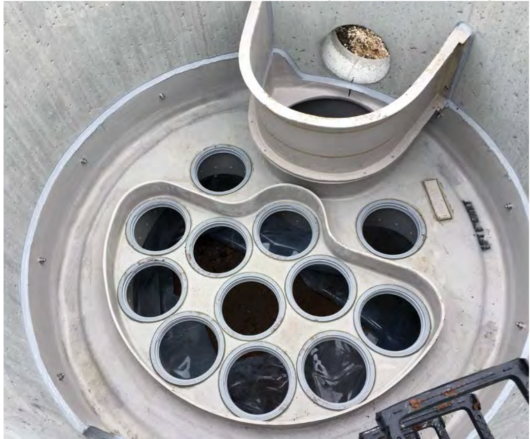
The pleated tentacles of the Jellyfish® Filter provide a large surface area for pollutant removal.
