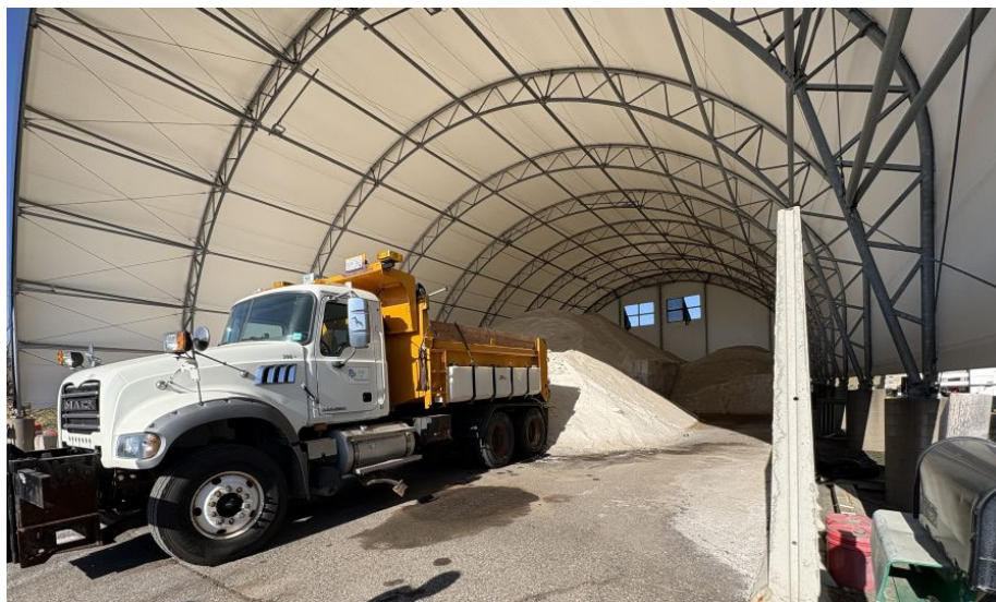
Plymouth salt storage building
