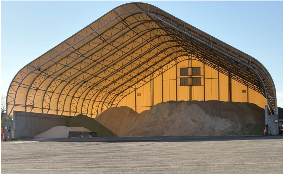
MnDOT salt storage building
