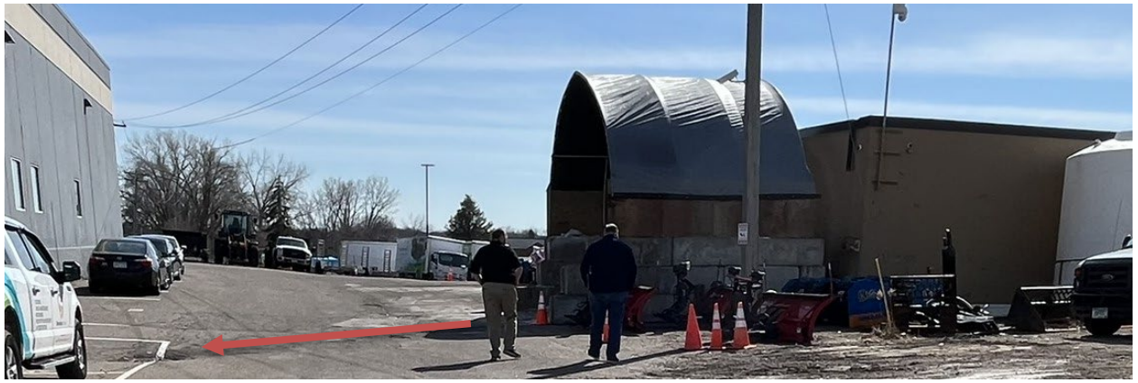
Drainage to storm sewer from salt shed
