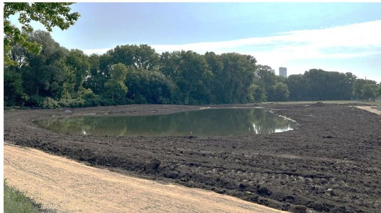
Construction of the ponds is complete and stormwater from the neighborhood to the west is not being routed through new storm sewers to the ponds. Some finishing work is underway such as cutting off and cleaning up pipe ends, final grading, seeding, etc. Project website: <http://www.bassettcreekwmo.org/projects/all-projects/bryn-mawr-meadows-water-quality-improvement-project>
