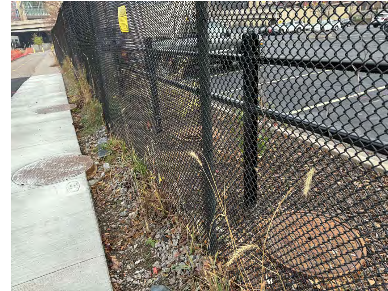
2 C-103 DETAIL: STA. 134+10 MAINTENANCE HOLE
