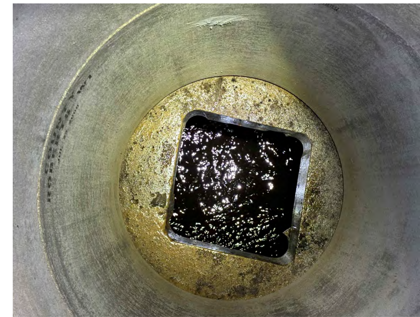
A C-104 DETAIL: STA. 129+10 MAINTENANCE HOLE INTERIOR
