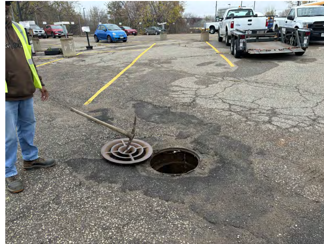
1 C-103 DETAIL: STA. 170+80 MAINTENANCE HOLE
