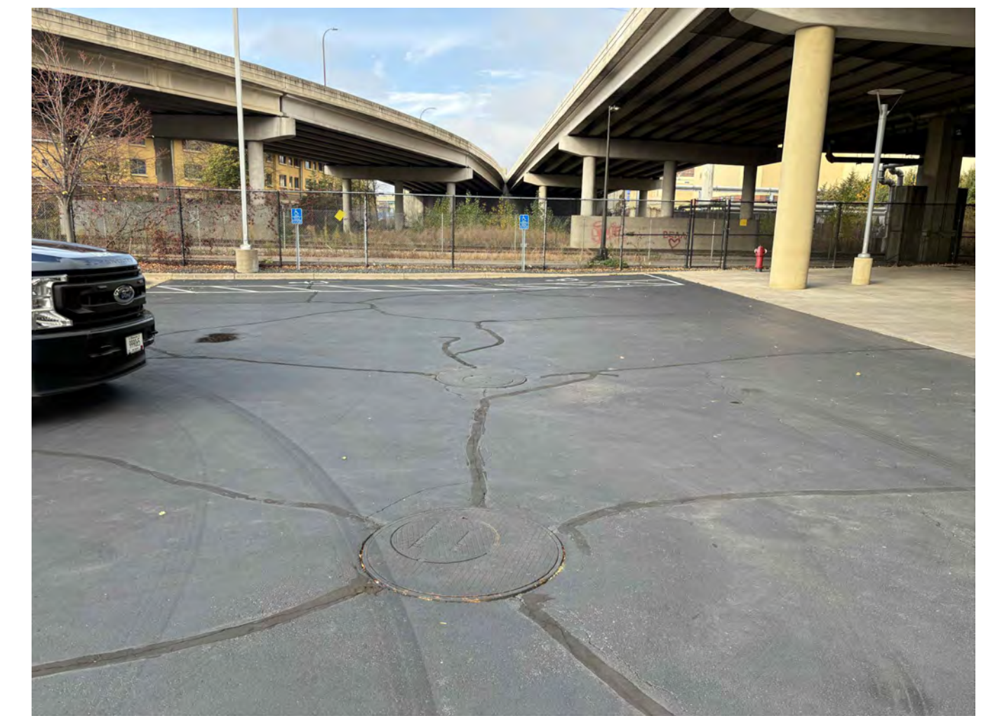
3 C-104 DETAIL: STA. 129+10 MAINTENANCE HOLE
