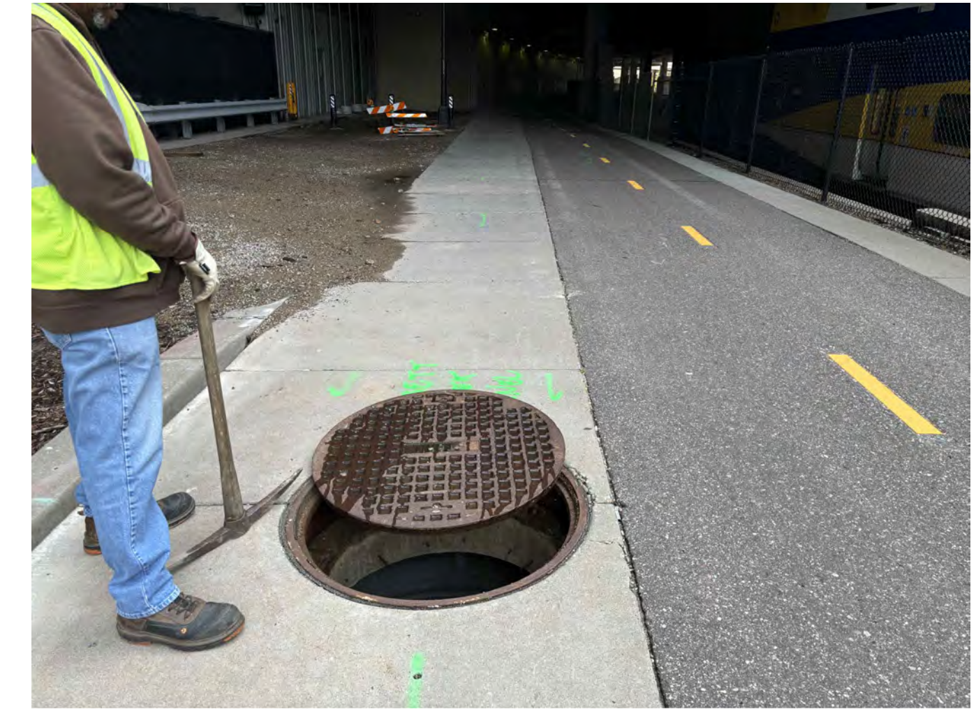
4 C-104 DETAIL: STA. 119+60 MAINTENANCE HOLE
