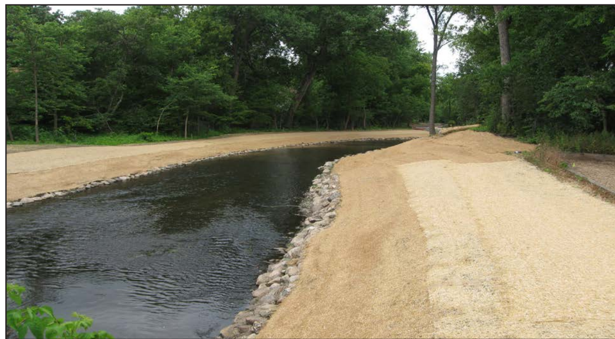
Bassett Creek restoration: bank stabilization and revegetation
