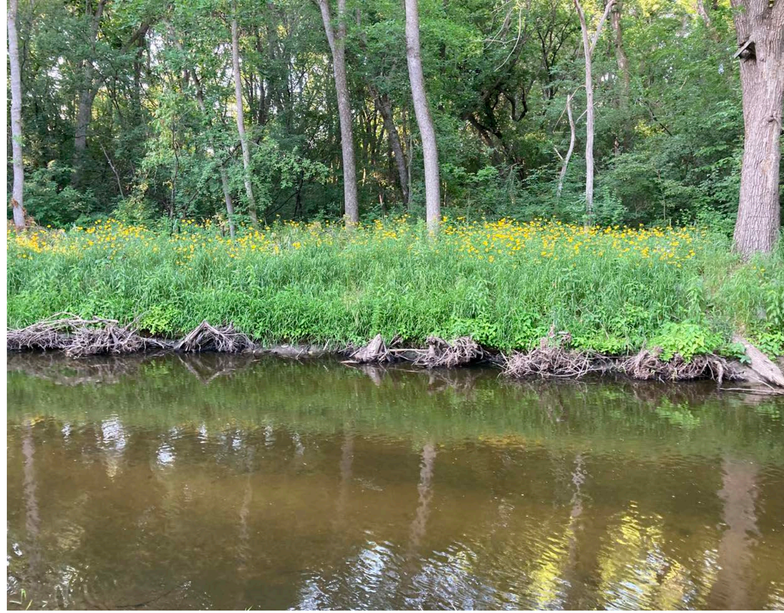
Toe Wood with VRSS and Grading
