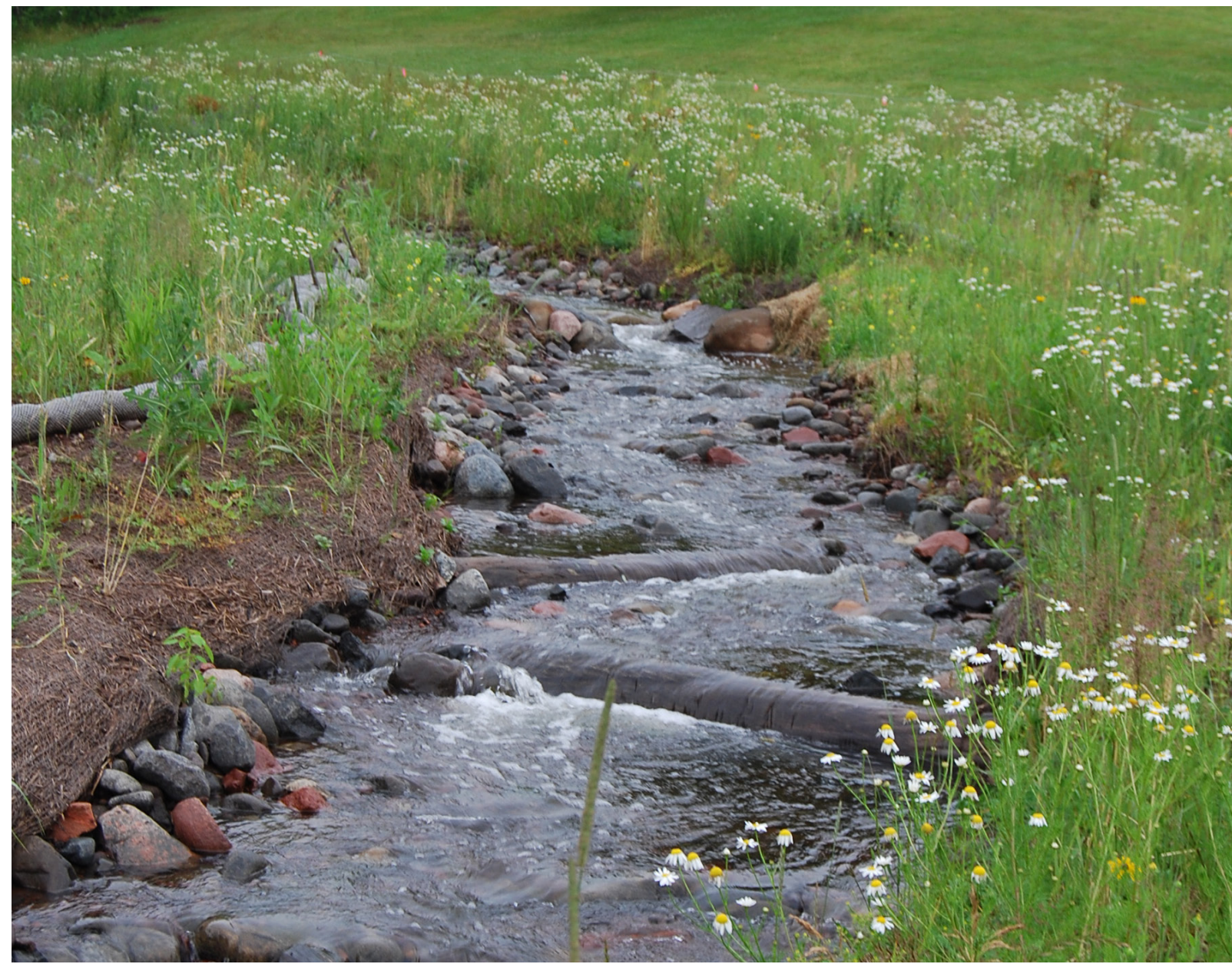
Rock Toe with Log Vanes
