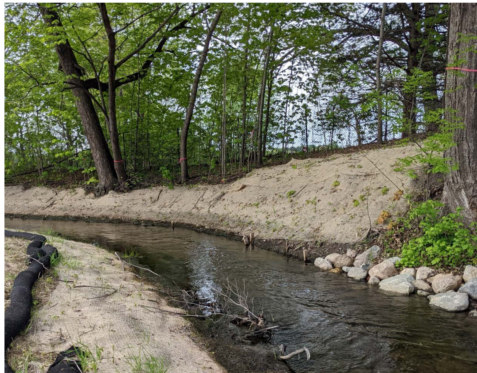
Coir Log with Bank Grading
