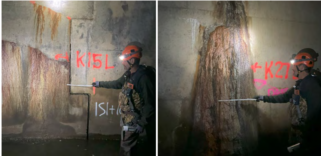
Figure 2 Typical Shear Keys Recommended for Repair
