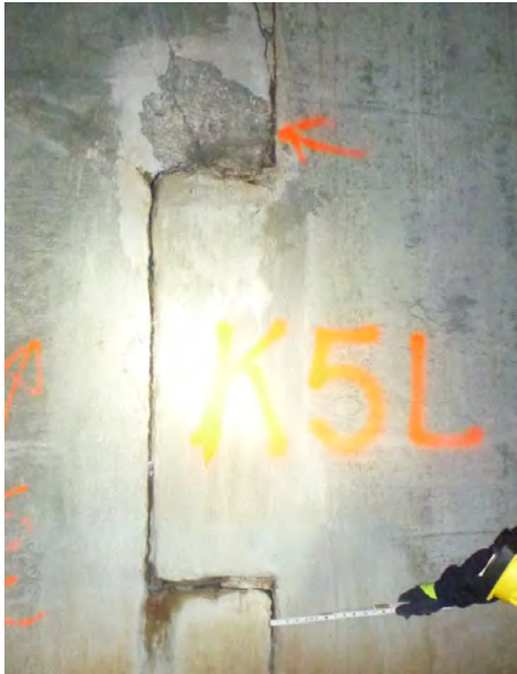
Figure 5 Typical Concrete Areas Recommended for Repair
