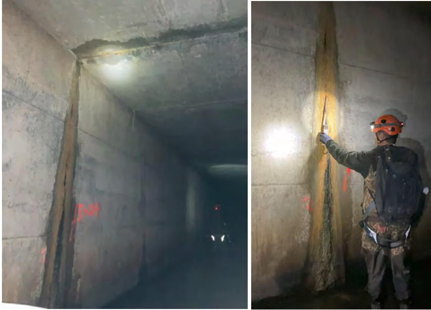
Figure 3 Typical Cracks Recommended for Repair
