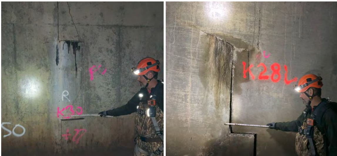
Figure 4 Typical Fractures Recommended for Repair
