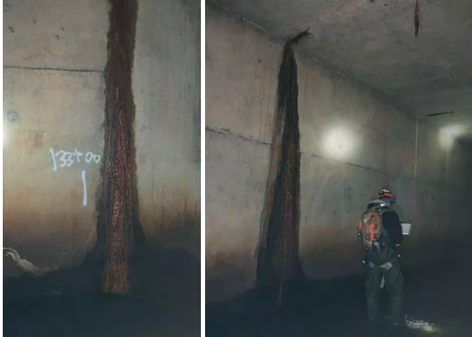
Figure 9 Typical Attached Deposits Recommended for Removal
