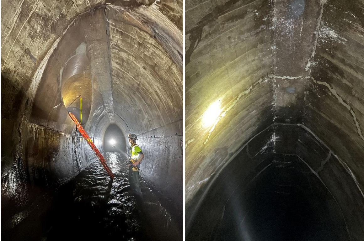
Figure 4: 3 rd Ave. Tunnel
