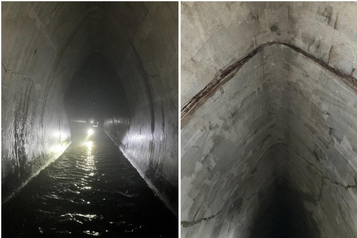
Figure 5: I-94/2 nd St. Tunnel
