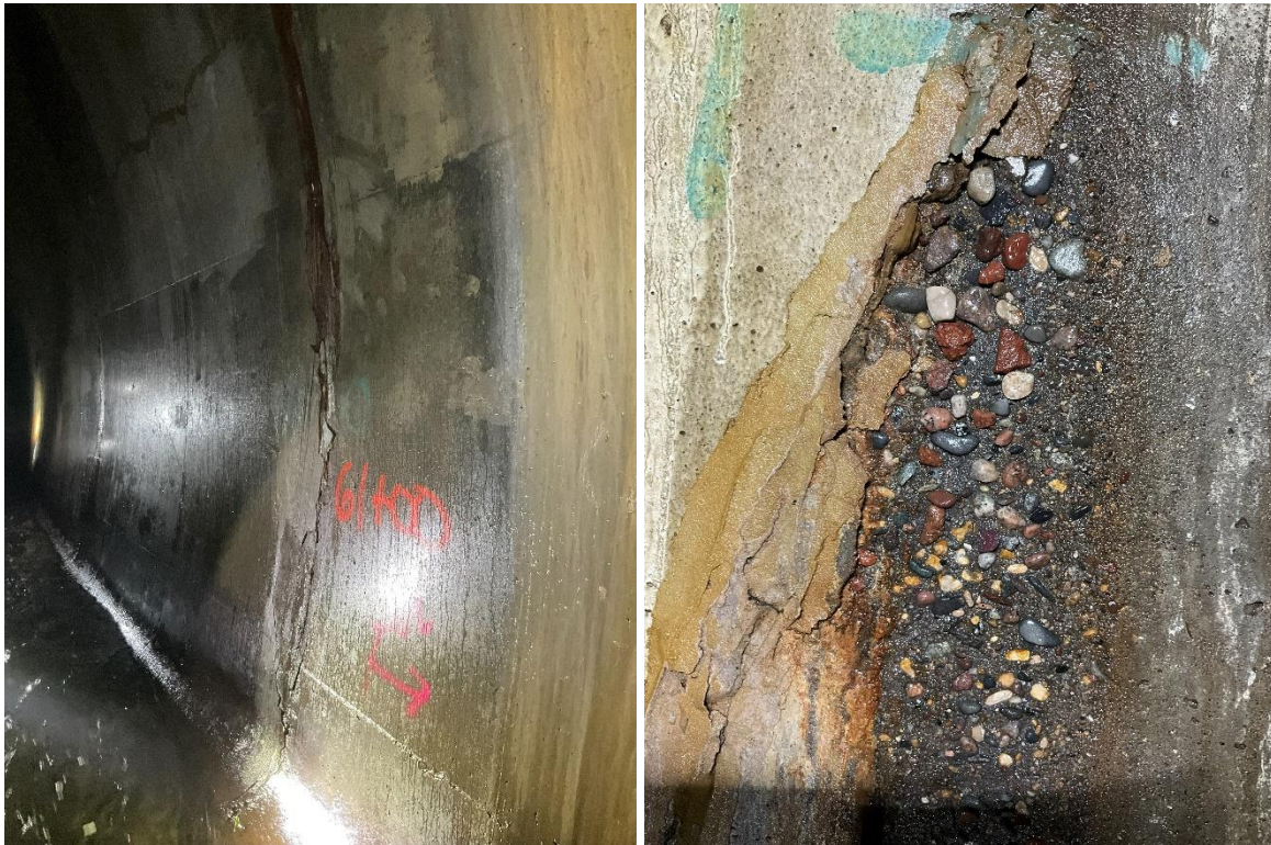
Figure 7: Location and closeup of new area of surface aggregate visible (SAV)
