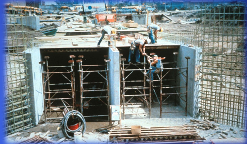
Double Box Culvert 1992
