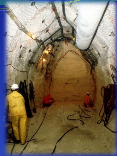
Third Ave. Tunnel 1990
