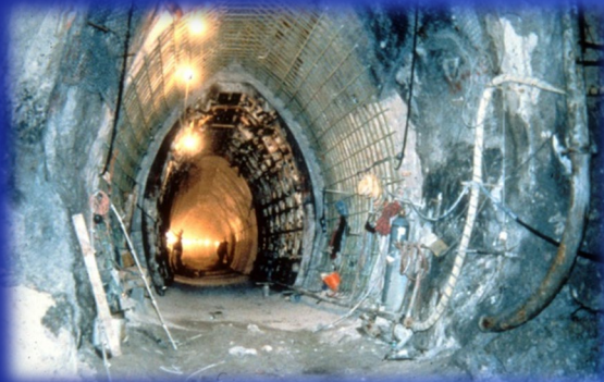
Second Street Tunnel 1978
