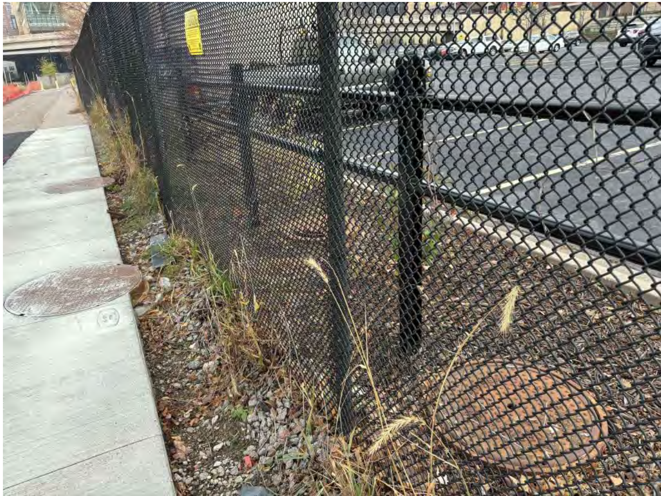
1 C-103 DETAIL: STA. 134+10 MAINTENANCE HOLE
