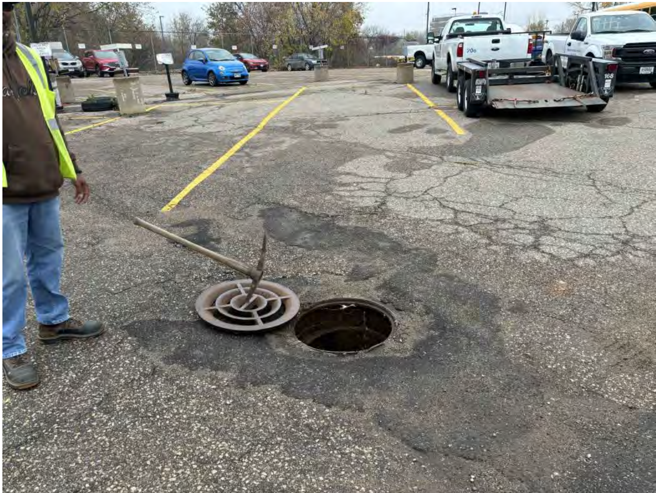
4 C-103 DETAIL: STA. 170+80 MAINTENANCE HOLE
