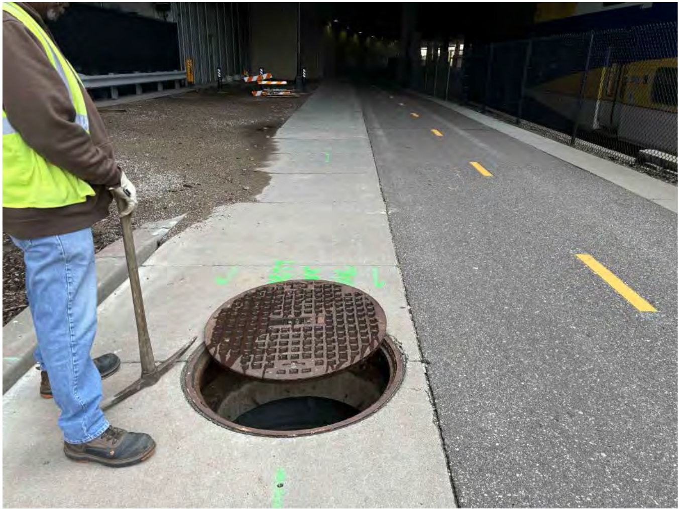
2 C-104 DETAIL: STA. 119+60 MAINTENANCE HOLE
