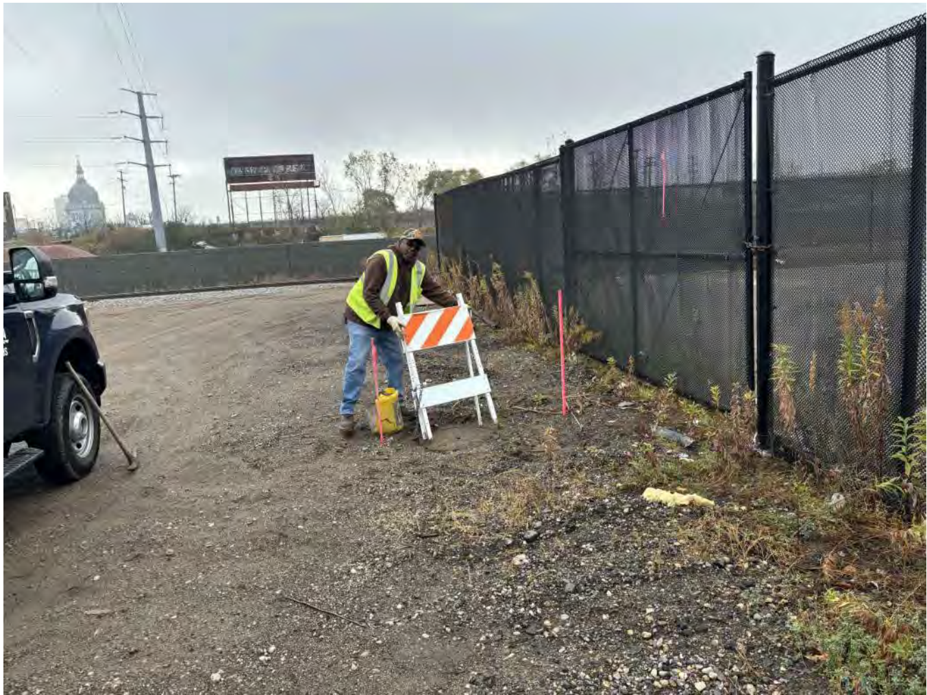
3 C-103 DETAIL: STA. 165+16 MAINTENANCE HOLE
