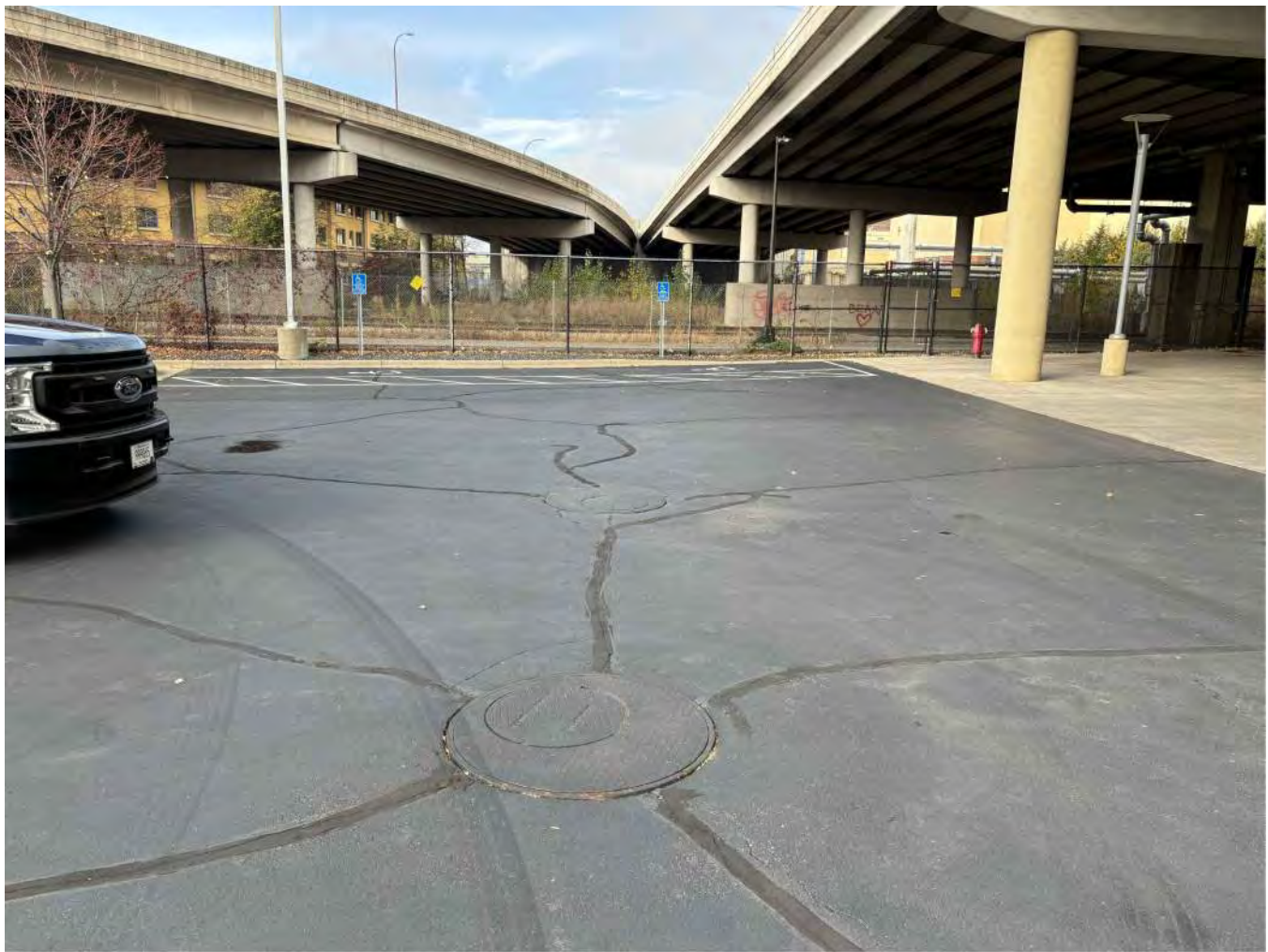
1 C-104 DETAIL: STA. 129+10 MAINTENANCE HOLE
