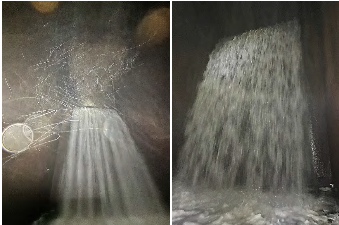
Figure 3: Drop Structure from Double Box Culvert to 3rd Ave. Tunnel (blurry due to heavy mist)
