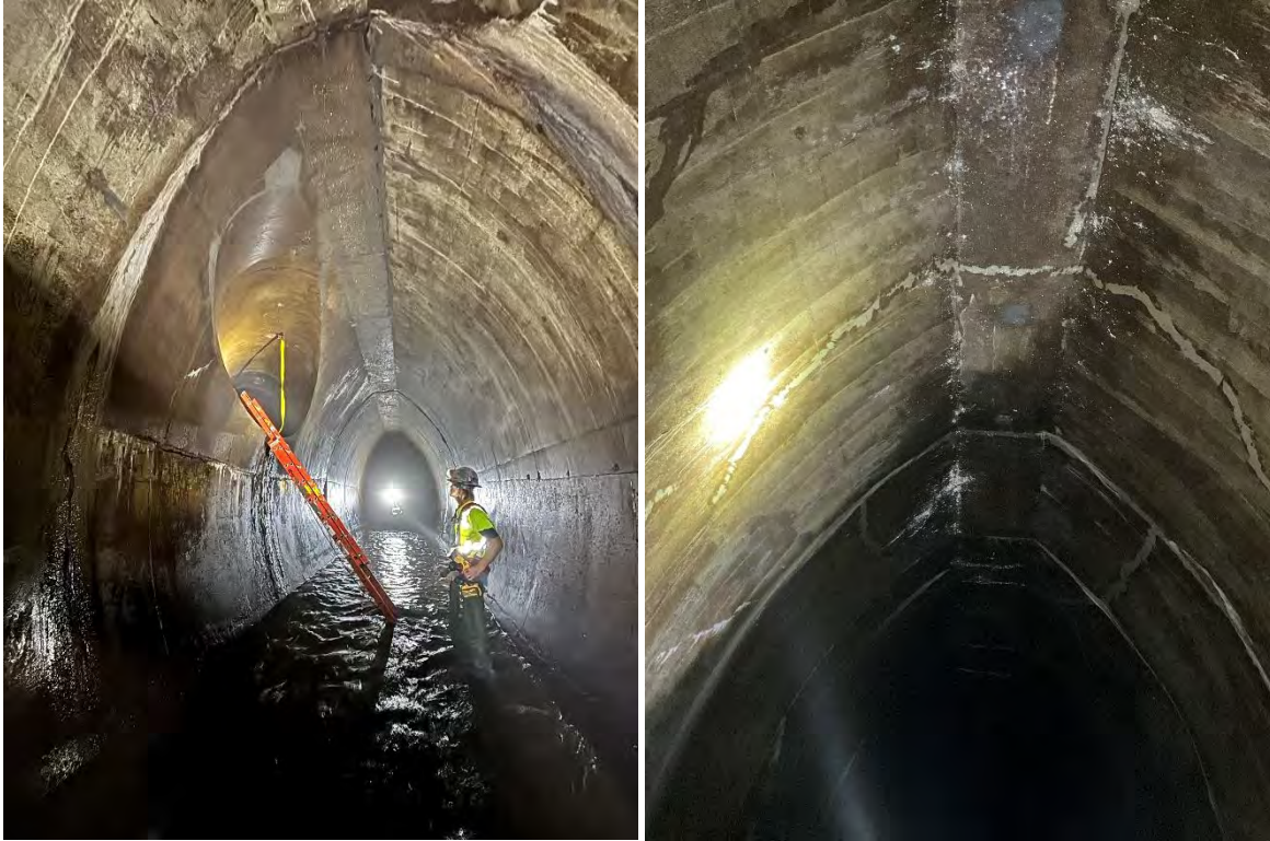
Figure 4: 3 rd Ave. Tunnel
