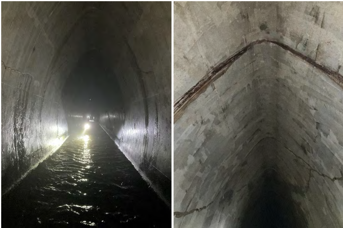
Figure 5: I-94/2 nd St. Tunnel
