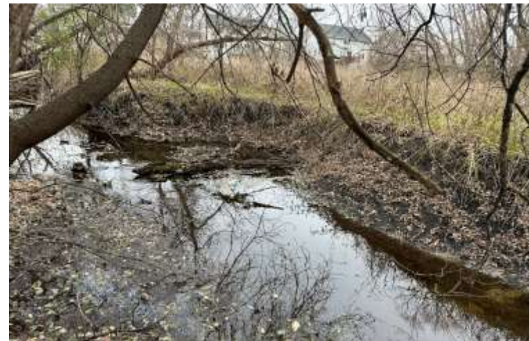
A section of eroding streambank along Ĥaĥá Wakpádaŋ / Main Stem of Bassett Creek evaluated in 2023 (Photo: Barr Engineering Co.).
